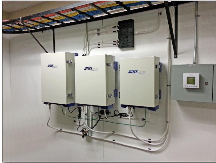
Example of repeaters installed in communications closet.
