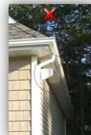
It is recommended that you mount your donor antenna in a spot that is free of any immediate obstructions. Making use of a pole or mounting bracket is recommended for optimum antenna performance.
